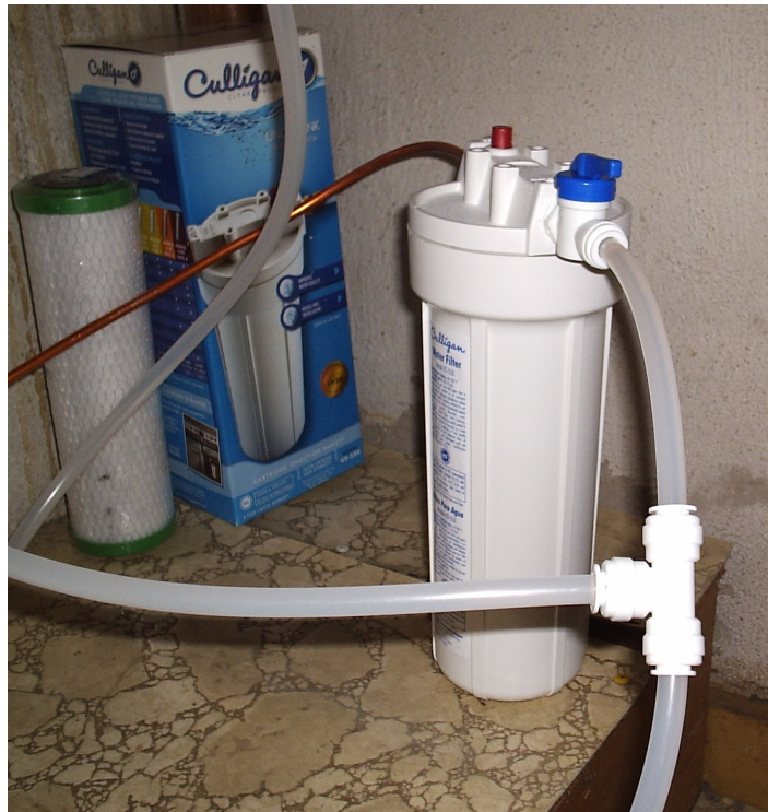
Present undersink style carbon drinking water filter.
